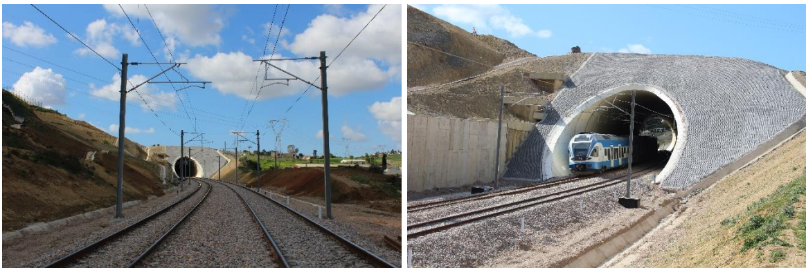
Figure 18. Tunnel en service
